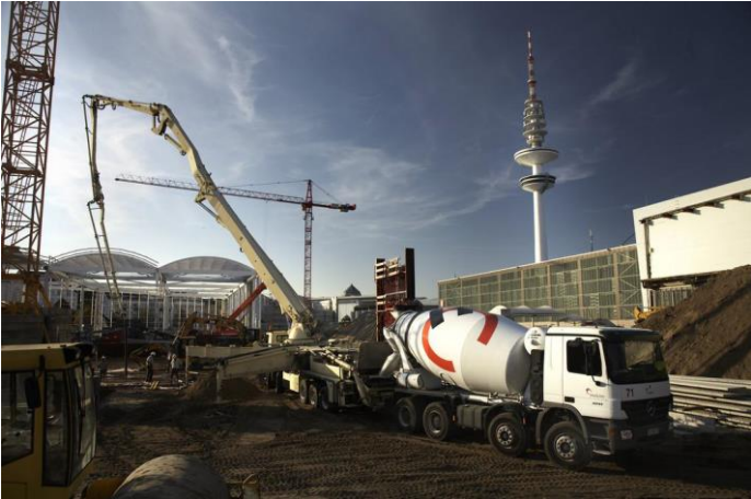
Figure B1: Mobile concrete pump
