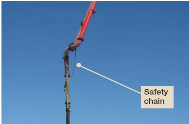
Figure 23: Discharge hose safety cable/chain
