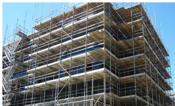
Figure 4: Example of good scaffolding with access stairs and edge protection all round
