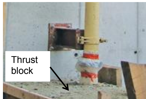
Figure 27: Thrust block
